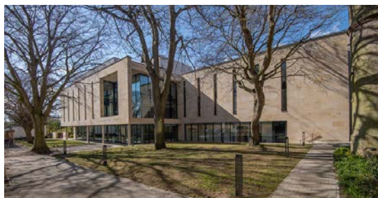
The Laidlaw Music Centre at the University of St Andrews.
